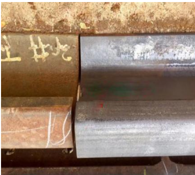
Rust removal on railway
