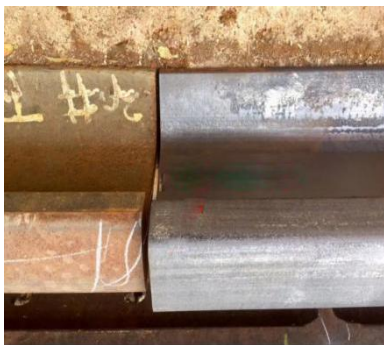
Rust removal on railway
